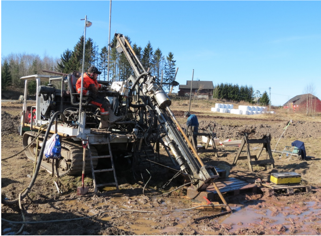
Diamantboring Nord with tracked mounted drill rig.
